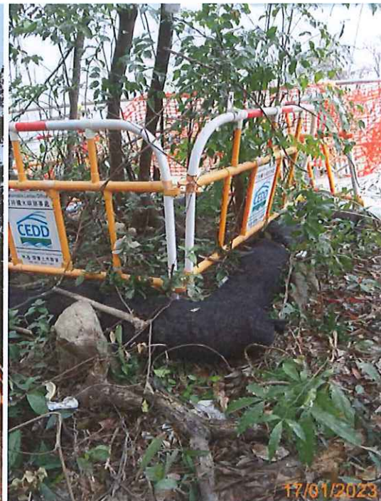
8: Protective fence sealed by sand bag
